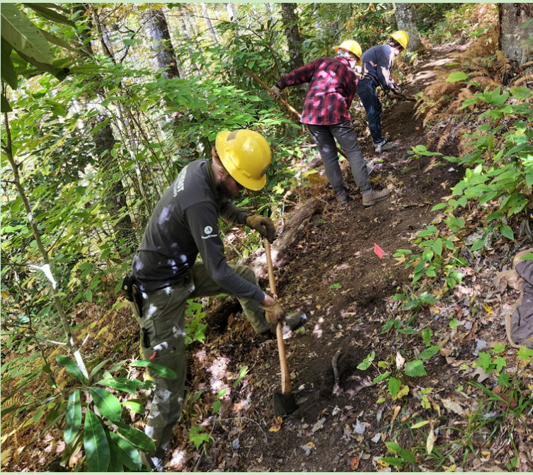
Members working on trail.
