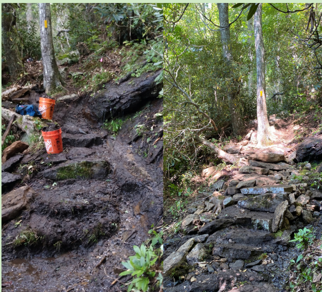
After and Before pic of stone stair case
