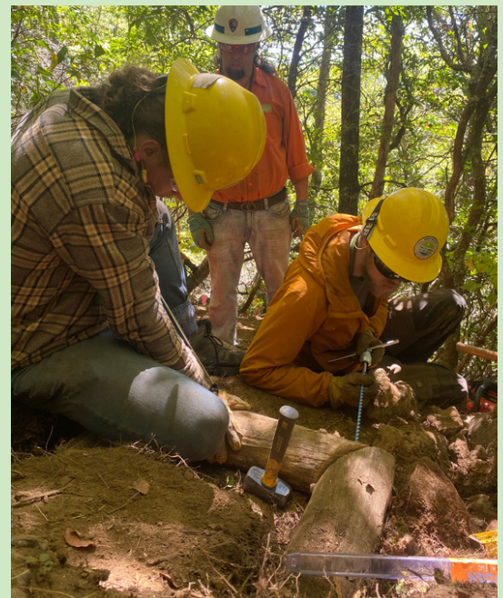
Members installing timber steps
