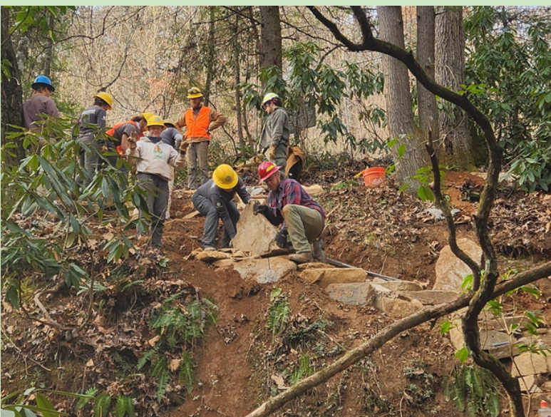
Crew working with partner staff to build stone staircase
